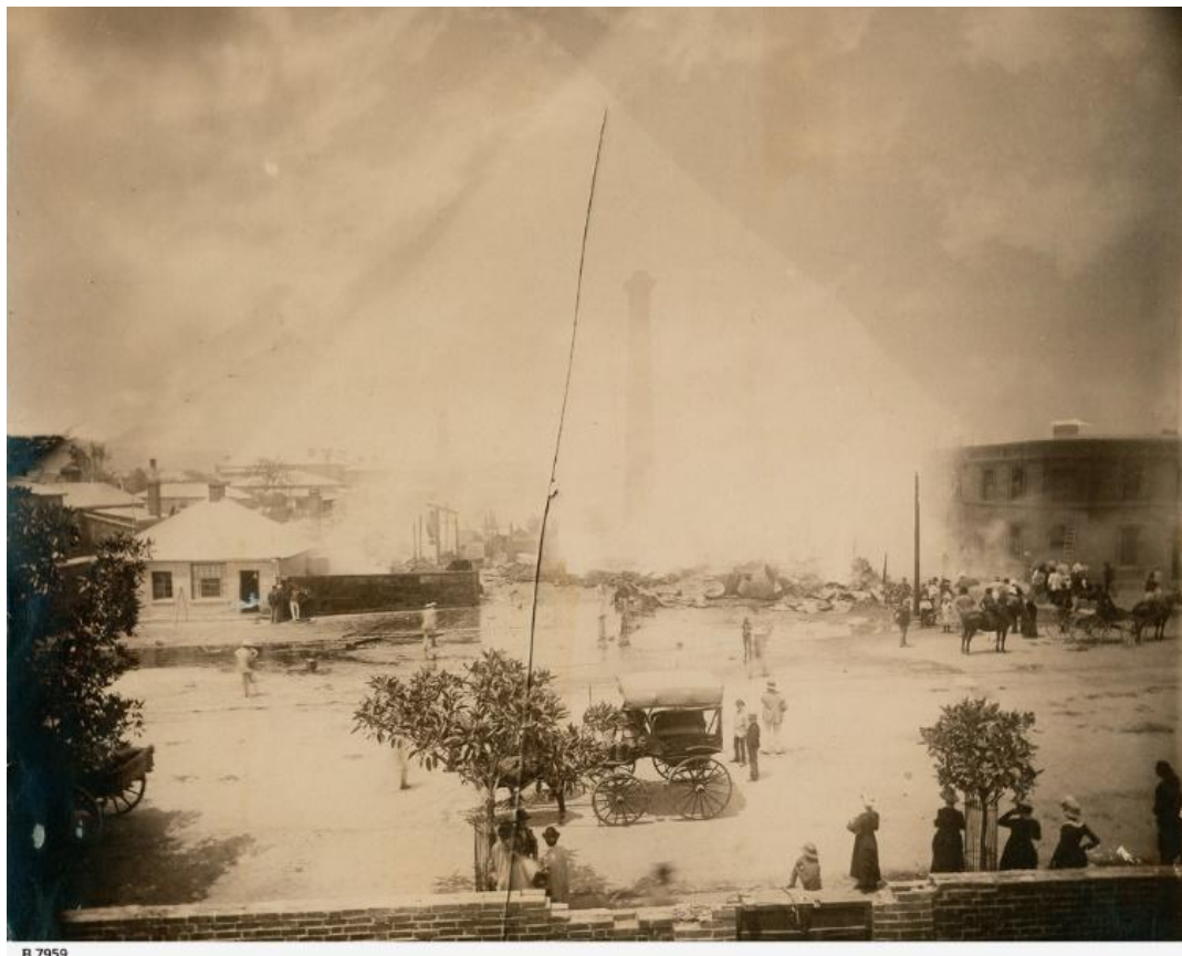
Grenfell Street [B 7959]. Grenfell Street, east end, after the fire at Burford's Soap factory. WH Burford and Son were soap and candle makers. The factory was on the corner of Grenfell Street and East Terrace. Residents complained about the smell from the soapworks and
